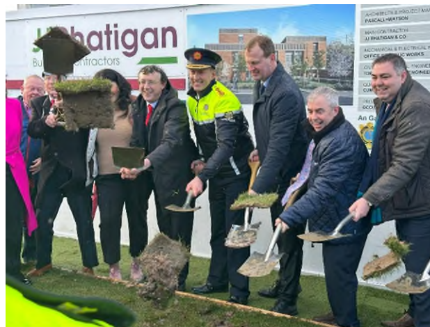
2Commissioner Kelly and Minister for Justice, Home Affairs and Migration, Jim O'Callaghan TD conducting the sod turning, together with Minister of State, Kevin Boxer Moran TD, Cllr Michael Looney, Cathaoirleach Macroom Municipal District, Senator Nicole R
