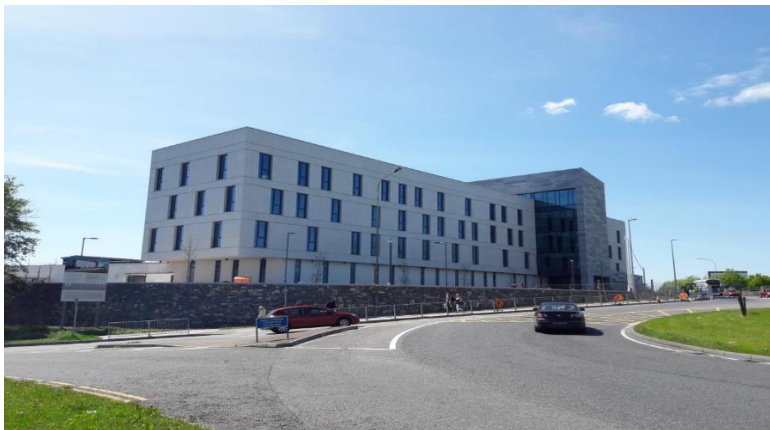
External view (eastern elevation)
