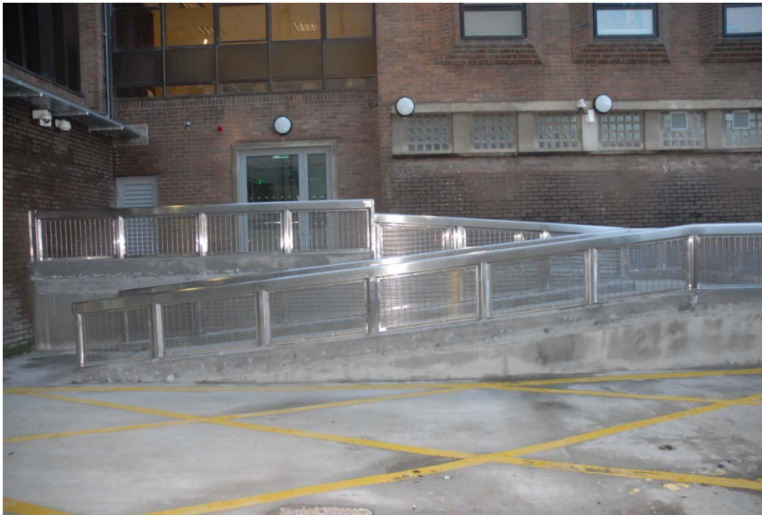
New Entrance to Custody Suite in rear yard
