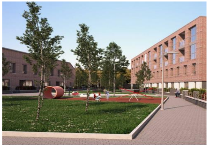
Dublin City Council housing estate to be built in Ballyfermot -
